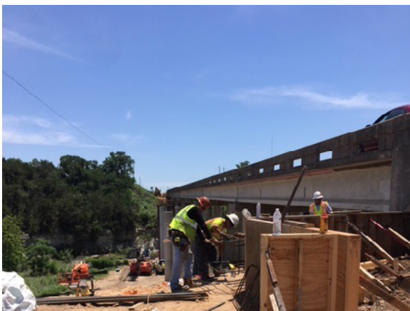
5. Sterling Forming Abutment N of Onion Crk Right
