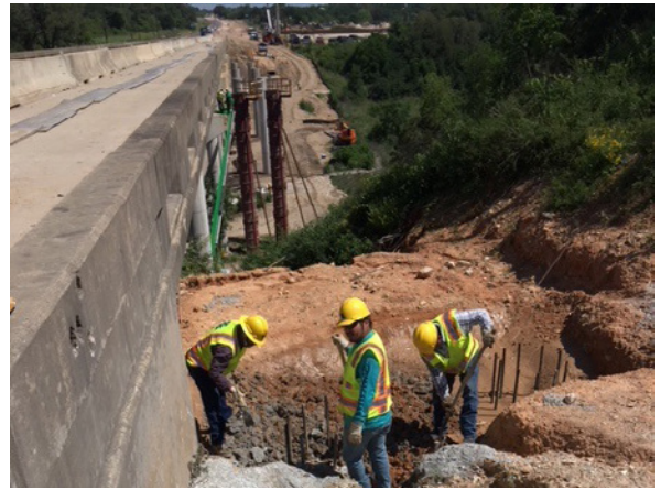
4. Sterling Forming Abutment N of Onion Crk Left
