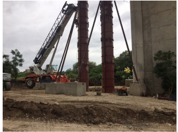
2. Sterling Pouring Columns at Onion Crk
