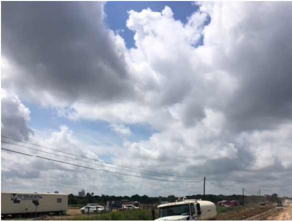
1. Sterling Earthwork Operations N of Onion Crk
