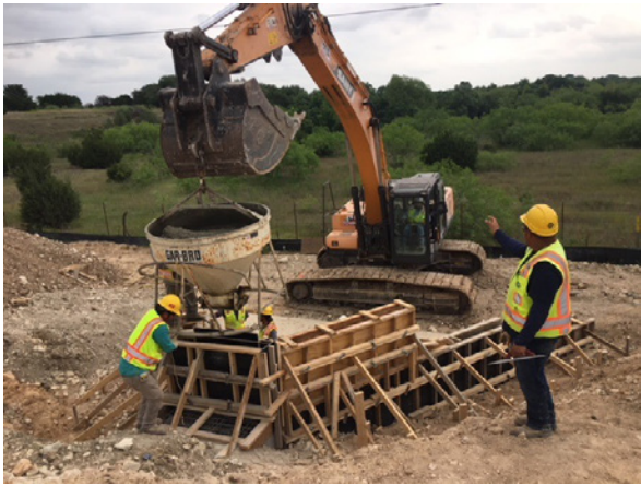
3. Sterling Pouring Headwall at Culvert 1 N of Mustang Crk
