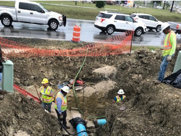
7. Sterling Completing Waterline Tie-in at RM 967z
