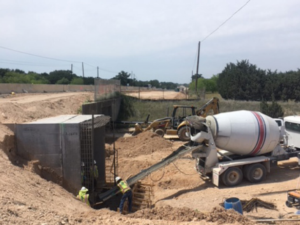
7. Sterling Pouring Footing a Truck Culvert N of Mustang Crk
