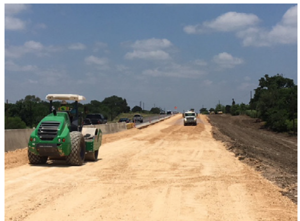
6. Sterling Placing Flexbase N of Mustang Crk
