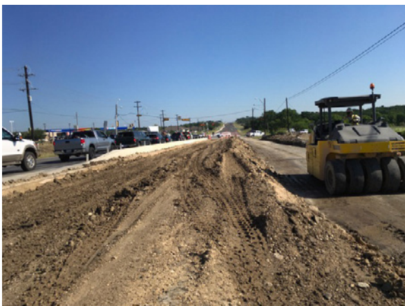
5. Sterling Earthwork Operations S of Rm 967
