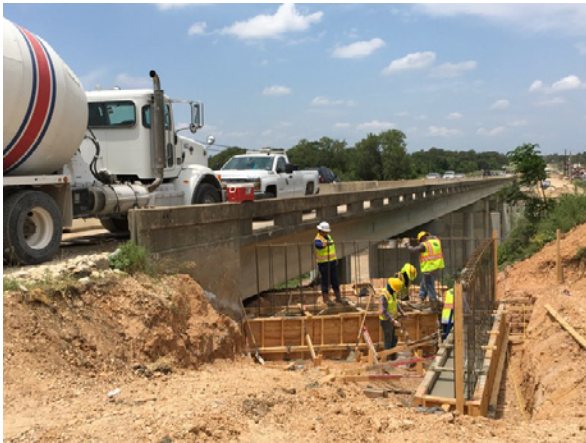
3. Sterling Pouring Abutment S of Onion Crk Right
