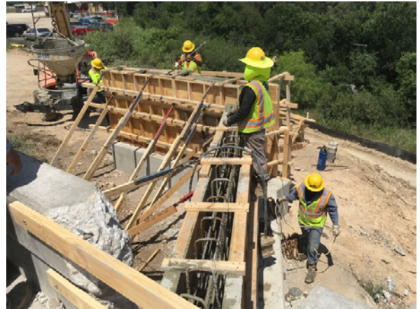
2. Sterling Pouring Abutment N of Onion Crk Right
