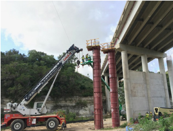
1. Sterling Forming Columns at Onion Crk
