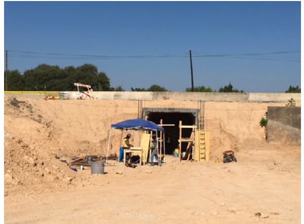
2. Sterling Forming Headwall at Truck Culvert N of Mustang Crk
