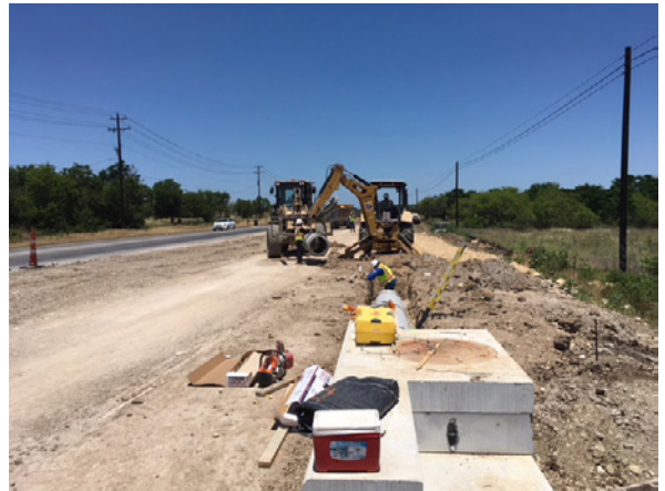
4. Sterling Installing RCP at Hy Rd Right Roadway
