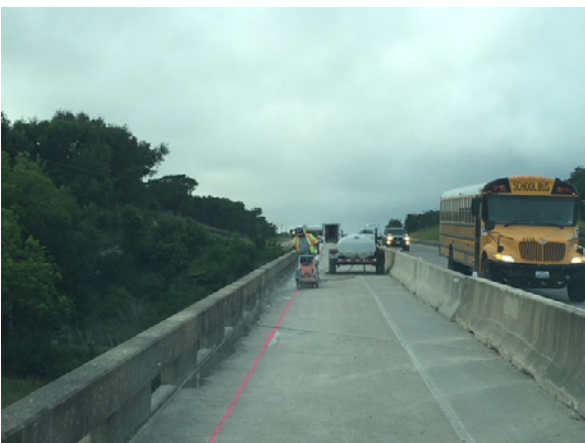
5. JR Ramon Sawcutting Onion Crk Bridge
