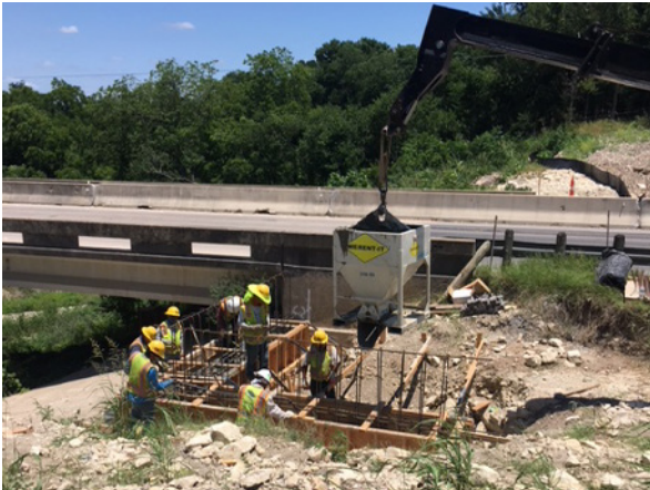
1. Sterling Pouring Abutment S of Mustang Crk Left
