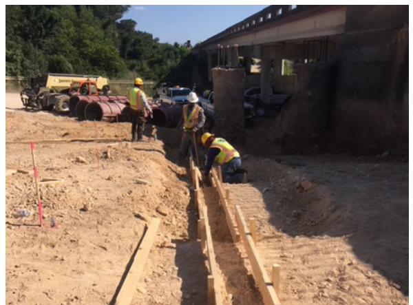
6. Sterling Digging Footing for MSE at Mustang Crk
