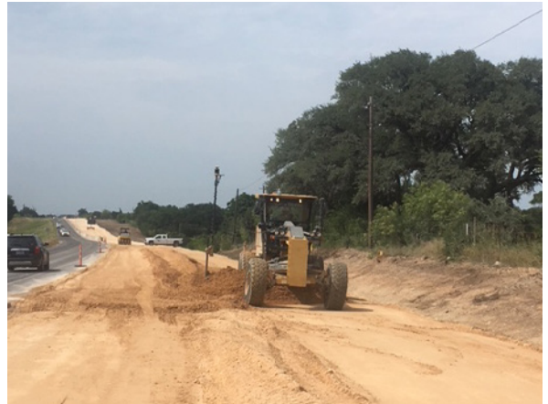
2. Sterling Placing Flexbase N of Mustang Crk
