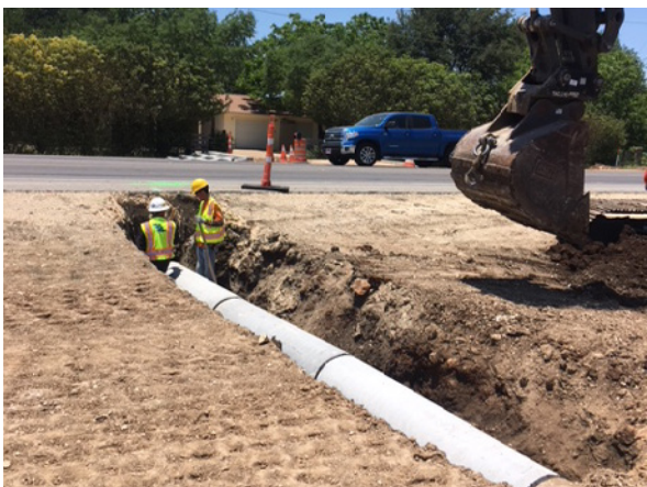
5. Sterling Installing RCP at Hy Rd Right Roadway
