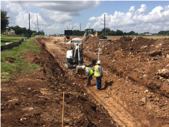
8. Rosch Digging Footing for Block Wall S of Oyster Creek
