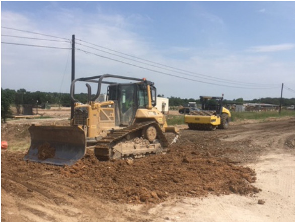
1. Sterling Earthwork Operations N of Onion Crk
