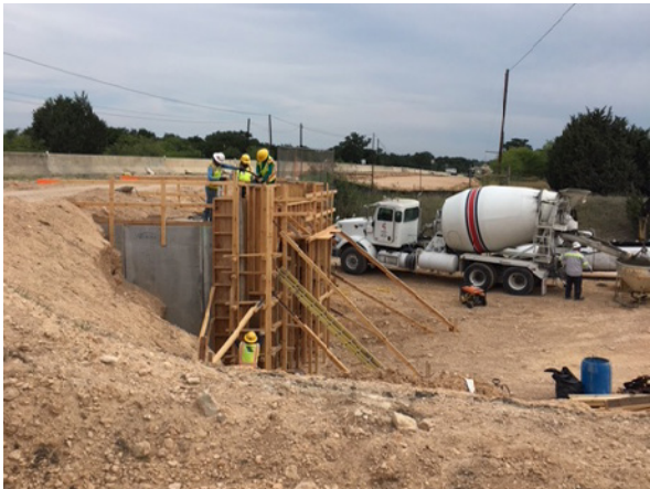
3. Sterling Forming Headwall at Truck Culvert N of Mustang Crk
