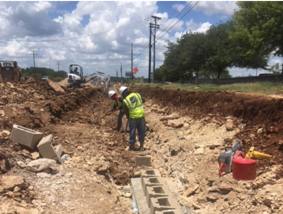
7. Rosch Beginning Block Wall Construction S of Oyster Crk
