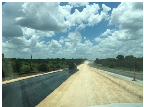
6. Austin Materials Placing Prime N of Mustang Crk
