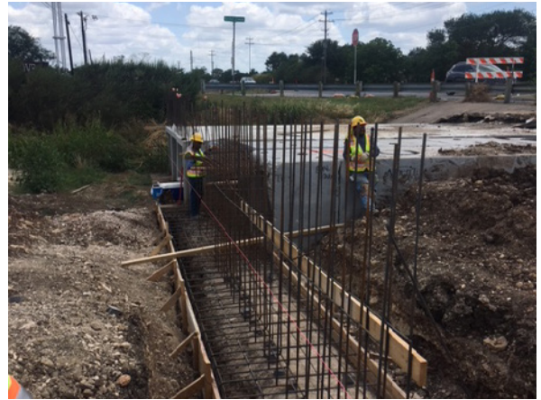
2. Sterling Forming Headwall at Culvert N of Oyster Crk
