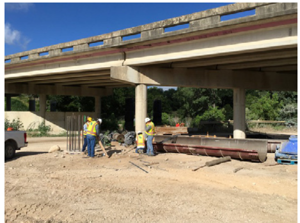
4. Sterling Forming Columns at Mustang Crk
