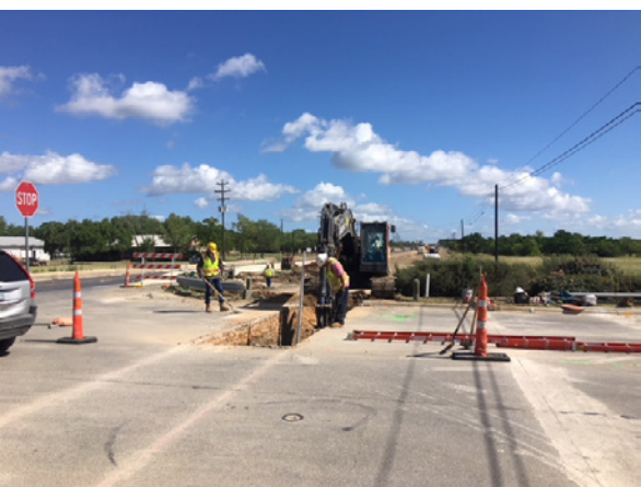
5. Sterling Installing RCP at Oyster Creek Right Roadway
