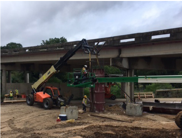
3. Sterling Pouring Columns at Mustang Crk
