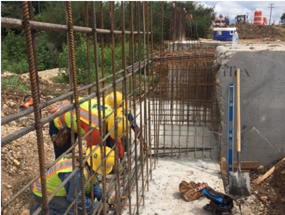
1. Sterling Constructing Headwall for Culvert N of Oyster Creek
