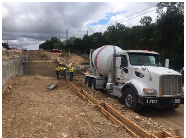
6. Sterling Pouring Footing for MSE at Onion Crk
