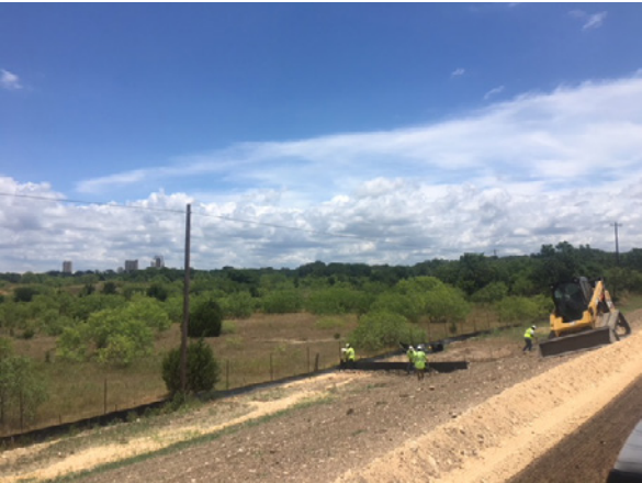
7. BMP Installing Erosion Control Device N of Mustang Crk
