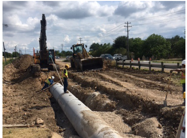
4. Sterling Installing RCP at S Oyster Creek Right Roadway
