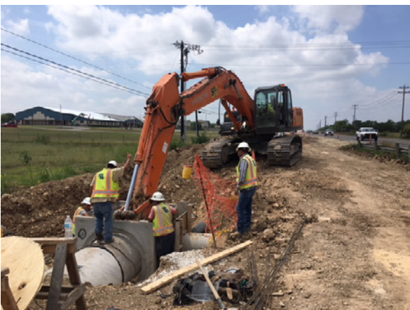
5. Sterling Installing RCP at S Oyster Creek Right Roadway
