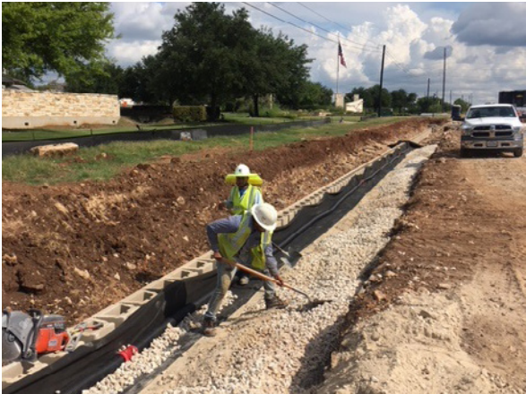
8. Rosch Constructing Block Wall Construction S of Oyster Crk
