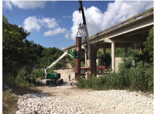
2. Sterling Forming Columns at Mustang Crk
