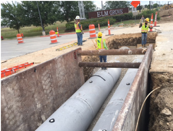
3. Sterling Installing RCP at Oyster Creek
