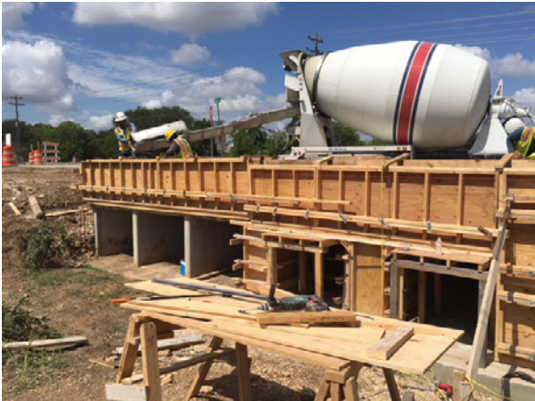
1. Sterling Forming Headwall for Culvert N of Oyster Creek
