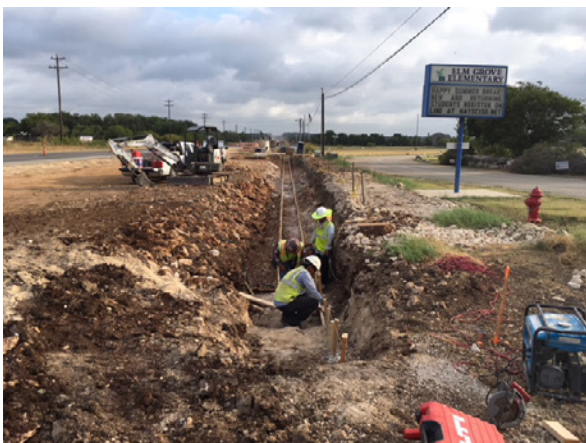
5. Rosch Constructing Block Wall Construction S of Oyster Crk
