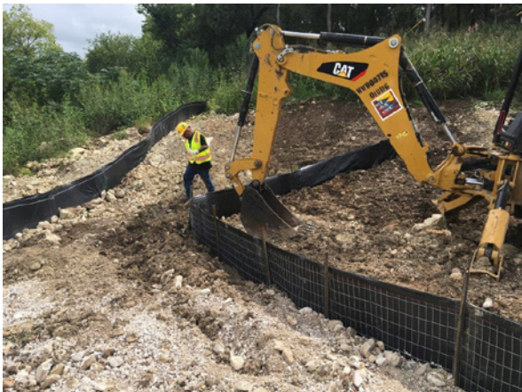
7. Sterling Performing Erosion Control
