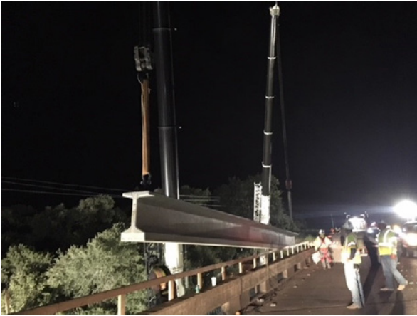
1. Sterling Placing Beams at Mustang Crk Bridge
