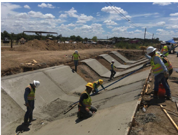
5. Sterling Pouring Riprap N of Onion Crk
