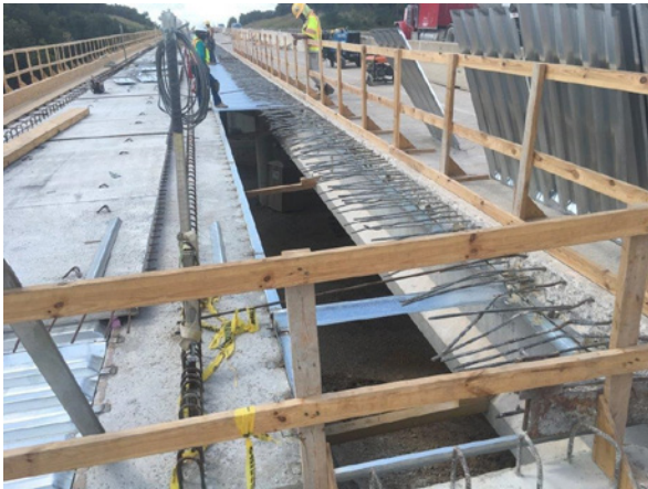
3. Sterling Installing Metal Decking at Mustang Crk Bridge
