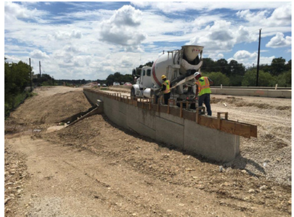
4. Sterling Constructing MSE Wall N of Onion Crk
