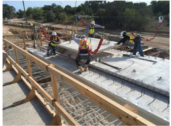
2. Sterling Placing Bridge Panels at Mustang Crk Bridge
