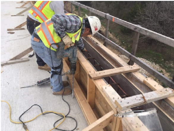
3. Macias Concrete Forming T401 Rail at Mustang Creek Bridge
