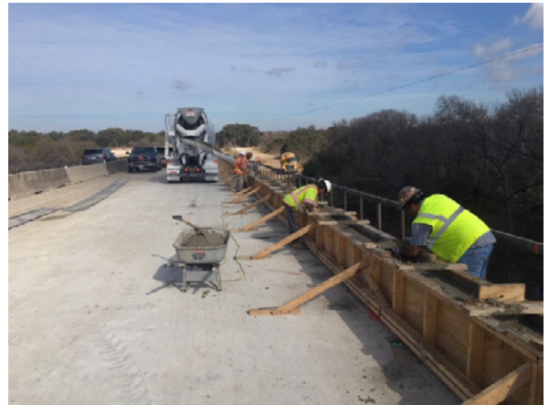
4. Macias Concrete Pouring T401 Rail at Mustang Creek Bridge
