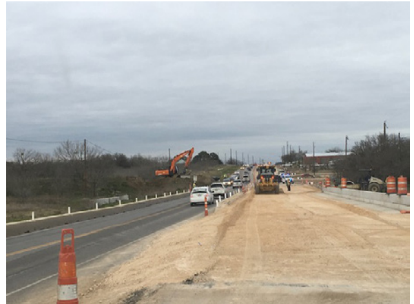
2. Sterling Placing Flexbase S of Cole Springs Rd
