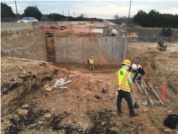
1. Sterling Constructing MSE Foundation at Centex
