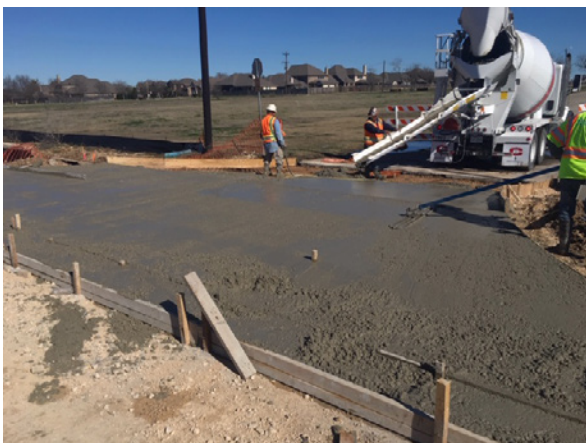
5. Macias Concrete Pouring Driveway at Elm Grove Elementary
