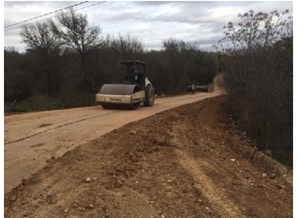
2. Sterling Constructing Driveway N of Onion Crk
