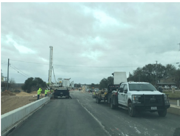
5. BMP Installing MBGF N of Onion Crk
