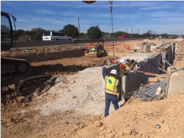
1. Sterling Constructing MSE Foundation at Centex
