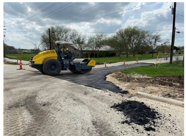
6. Sterling Side Street Construction at Hy Rd
