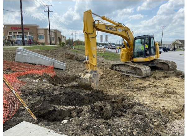
2. Sterling Performing Earthwork Operations S of RM 967
