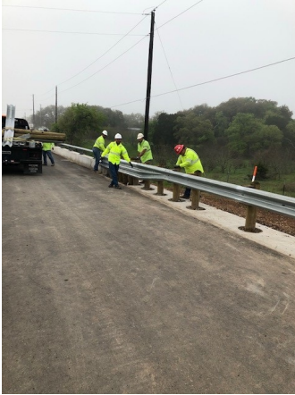
1. BMP Installing MBGF N of Onion Crk
