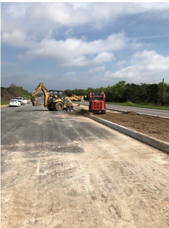
3. Sterling Placing Topsoil at Median S of Mustang Crk
