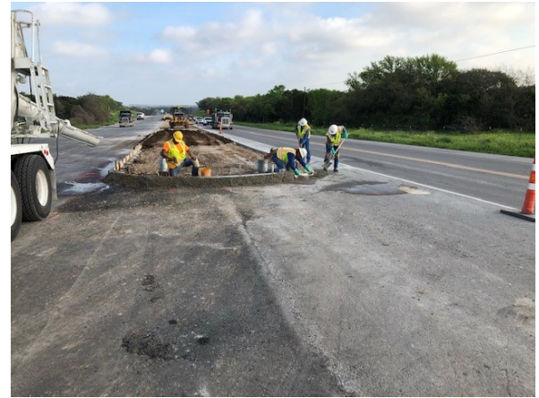
4. Sterling Pouring Median Curb S of Mustang Crk
